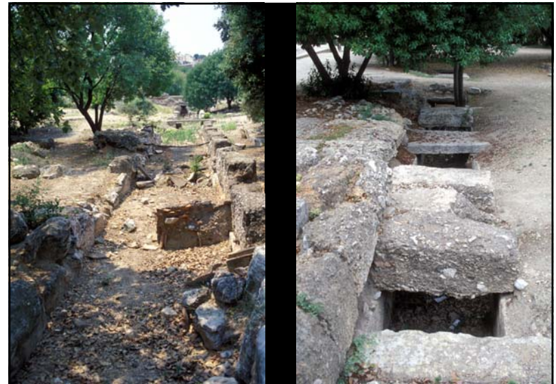
Storm drainage channels at the Agora, Athens, Greece
