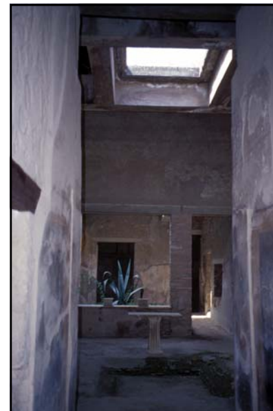
Impluvium (indoor pool and cistern for rain water storage), Pompeii, Italy (before 79 AD)
