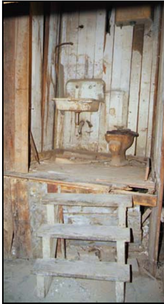
Elevated toilet to keep above hydraulic grade line during high tides, Seattle, WA (Underground Seattle Museum)
