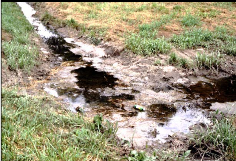
Upwelling sewage from broken sewer in backyard, Birmingham
