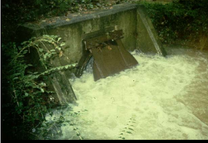
Sanitary Sewer Overflow, 5-Mile Creek, Birmingham, AL
