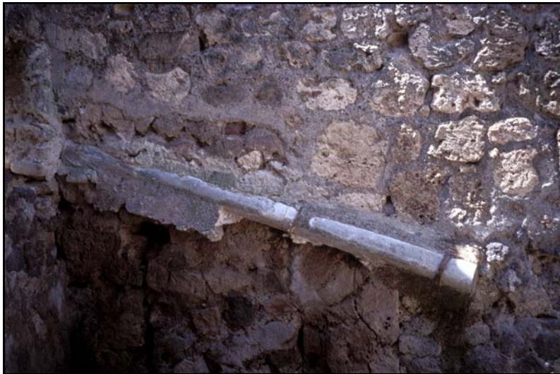
Pipe at Pompeii, Italy (before 79 AD)
